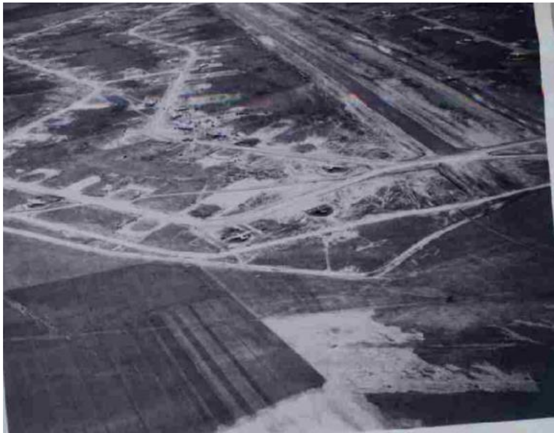
Hardstands and runway, looking west.
