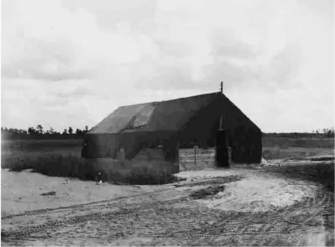
First Group Operations Building, AAB, Pine Castle, Florida, 20 September 43
