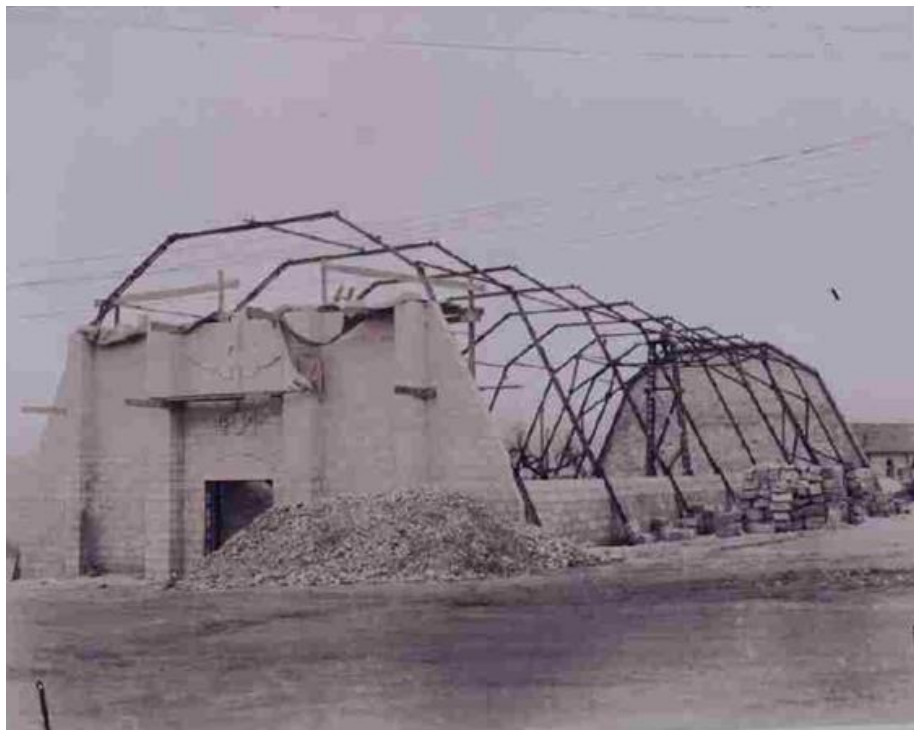
"Group Theatre and Gymnasium" Operations are proceeding according to plan.
