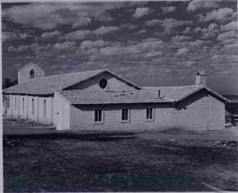
Rear view of Chapel showing office and reading room.
