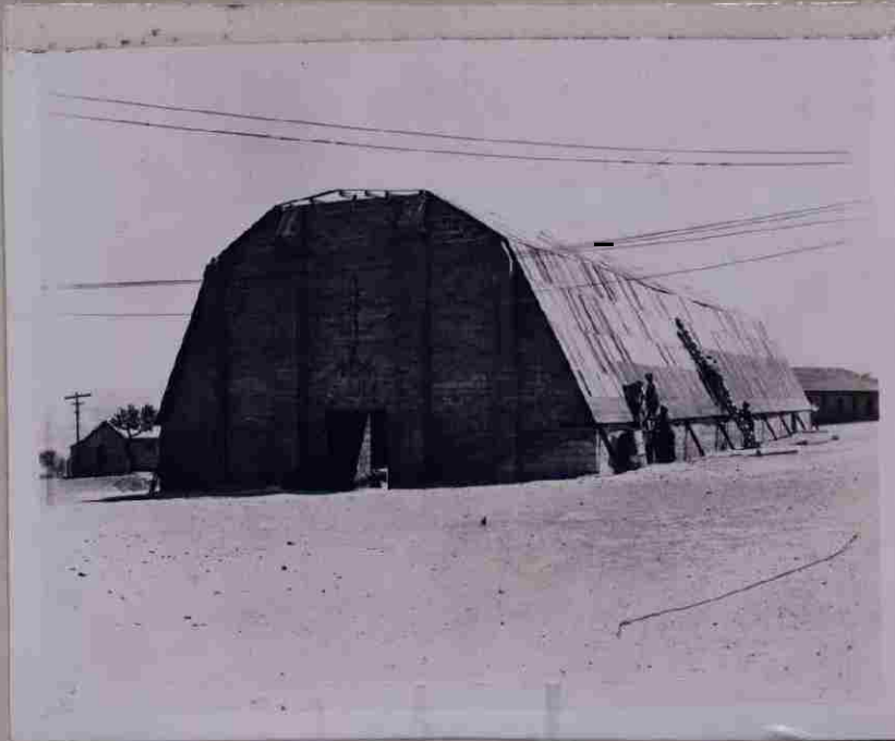
Group Theater nears completion.
