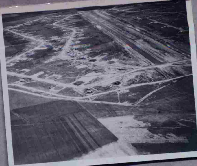
Hardstands and Runway, looking west.
